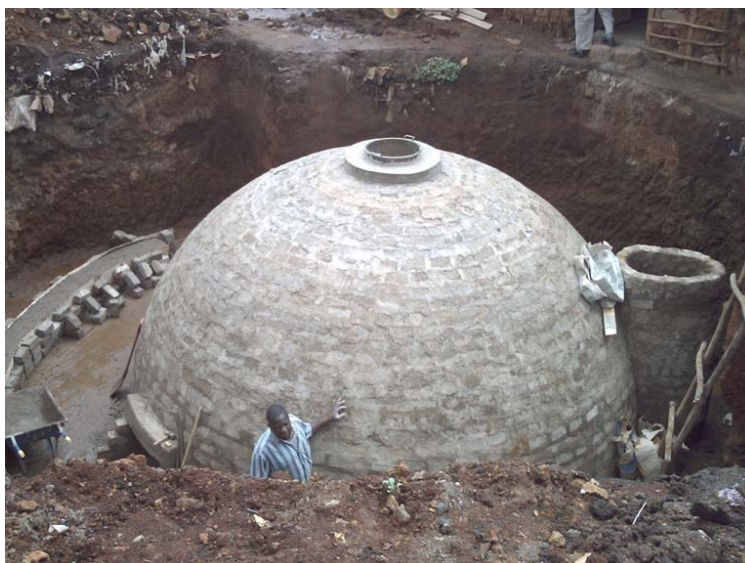
Figure 3.14: Community-managed sanitation block in Gatwekera village, Kibera, Nairobi – top: the ground floor is the sanitation compartment with toilets, showers, clothes-washing facilities; and the top floor has a ‘community room’ used for meetings, weddings, parties, etc. and a small kitchen; bottom: underneath the ground floor is a large anaerobic digester which receives all the wastewater from the sanitation block; the biogas generated in the digester is used for cooking in the kitchen on the top floor.
