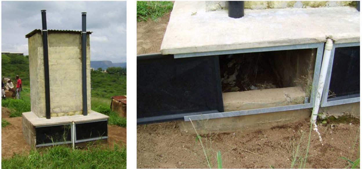
Figure 3.4: An eThekweni latrine – top left: front view showing the urine-diverting pedestal seat unit, urinal, and cover over the entrance to the vault not in use; top right: close-up of the urine-diverting pedestal seat unit; bottom left: rear view showing the two vent pipes (one for each vault) and the small urine pipe (in the centre) which leads to an adjacent soakaway; bottom right: close-up of one of the two vaults with the sliding door open showing the dehydrating vault contents.
