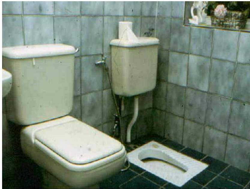
Figure 3.15: The toilet in a house in Bradford, England, belonging to an Asian doctor who has some family members and friends who are sitters and some who are squatters, so he installed both a pedestal-seat unit and a squat-pan unit. Notice the flexible water pipe and tap between the two units and the toilet paper on top of the squat-pan cistern – provision for both washers and wipers.
