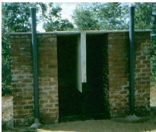
Figure 3.16: Double-compartment VIP latrine at a rural school in Zimbabwe: one side for girls, the other for boys.
