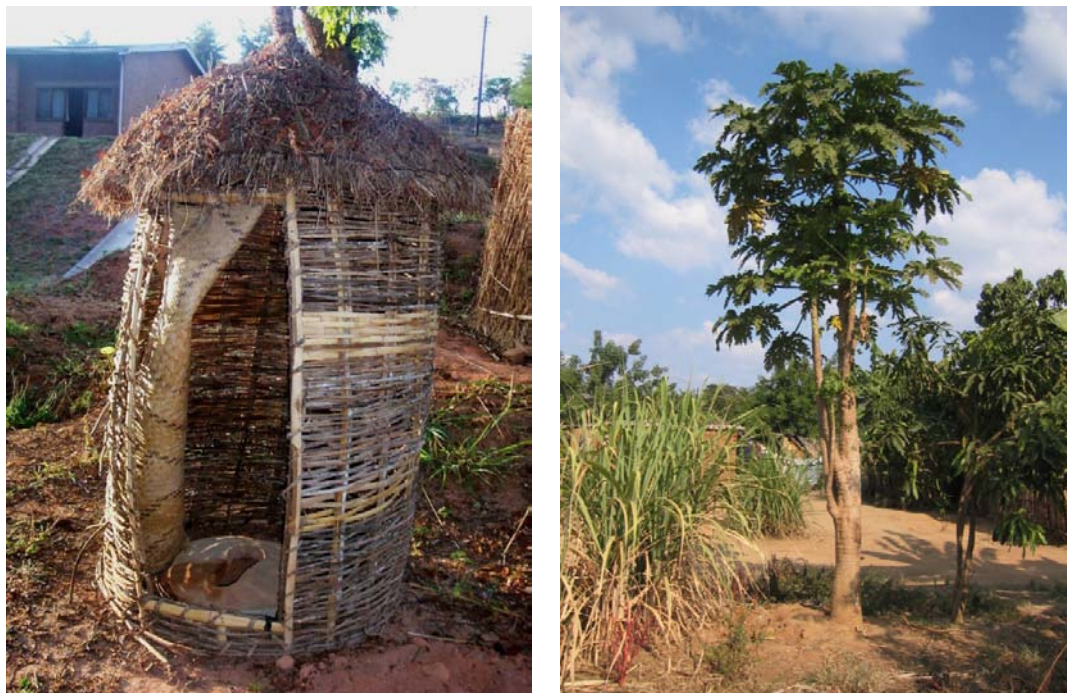
Figure 3.1: The Arborloo – top: schematic diagram; bottom left: a simple Arborloo superstructure; and bottom right: a papaya tree planted in a full Arborloo pit.
