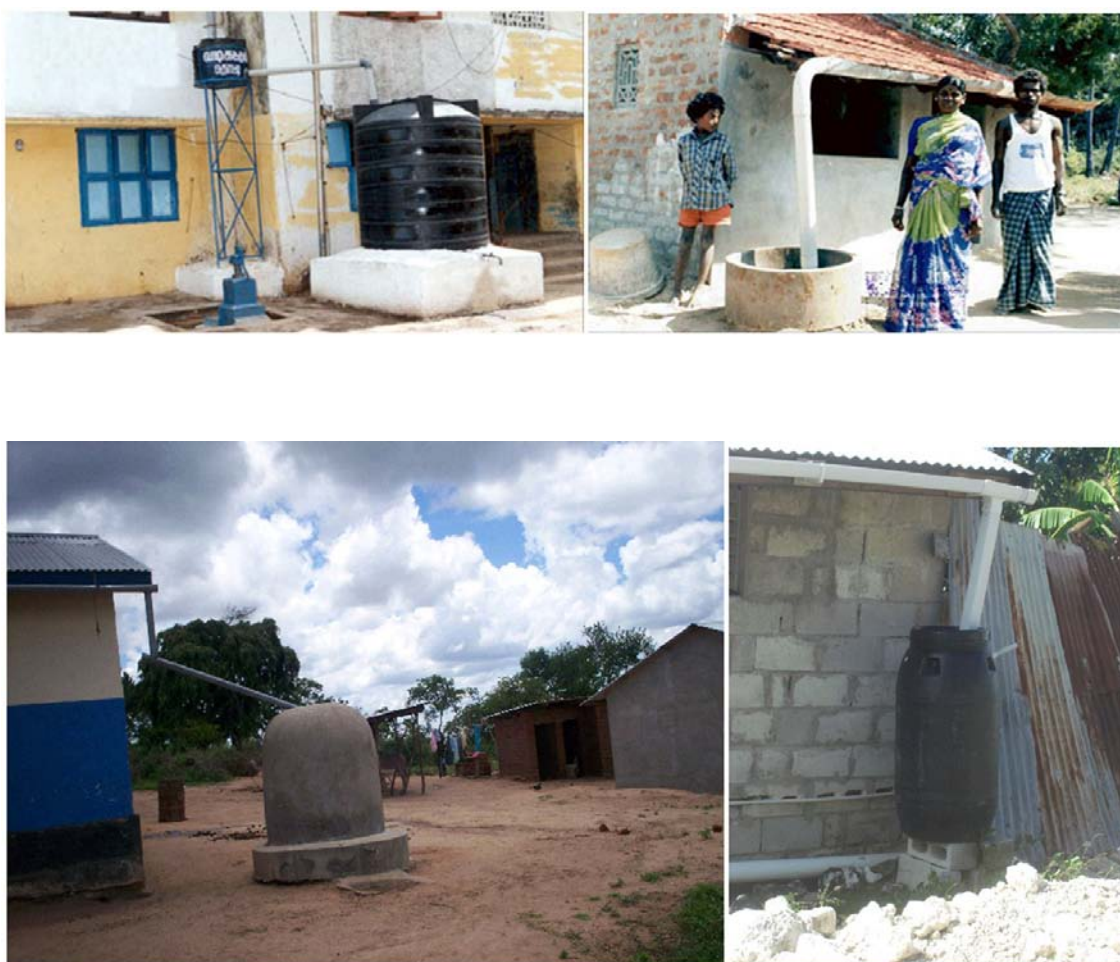
Figure 4.2: Rainwater harvesting from rooftops in Chennai India (12) and Kenya (13) A variety of materials can be used to store the collected water. Plastic vessels are often available in the local market and are light to transport and generally fairly cheap. Where these are not available, in-situ construction using light-weight ferro-cement is a good alternative. Underground tanks may be preferred in some locations due to greater storage capacity and the fact that water supplies tend to remain cooler.
