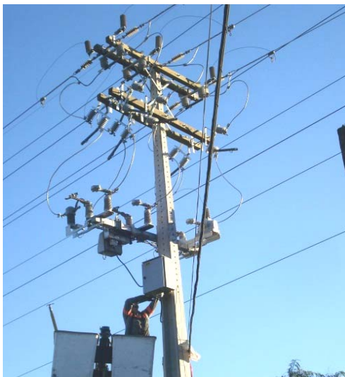
Fig. 8. Installation of a remote controlled switch.
